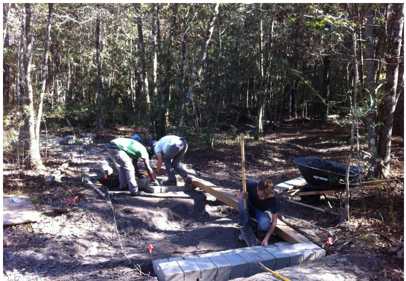
Figure 5: Installation of prefab. bridge foundations
